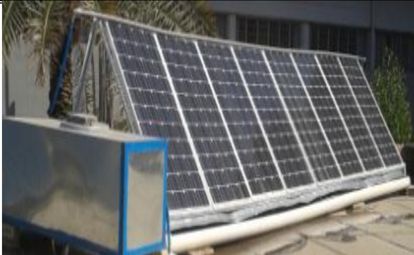
Figure(6) Using water pipe to clean the solar panels
