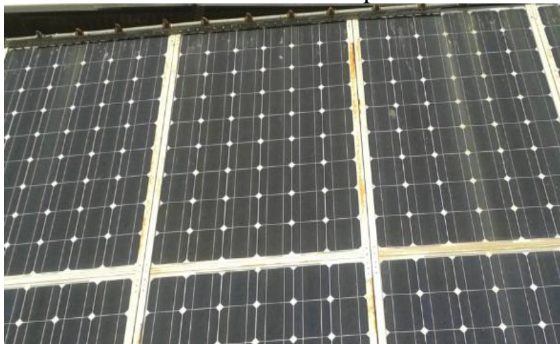
Figure(5) Using nozzles to clean the solar panels
