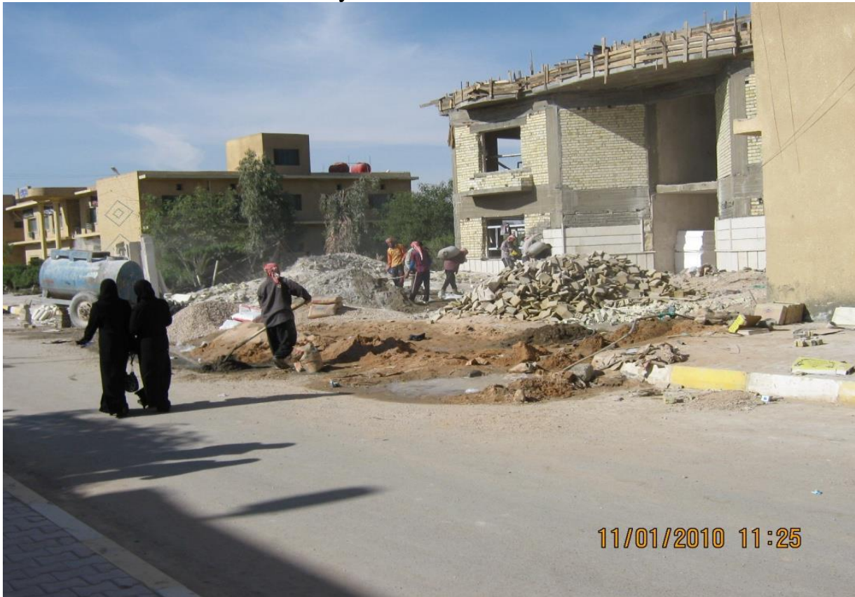
Figure 1: construction site at Karbala University (old campus)
